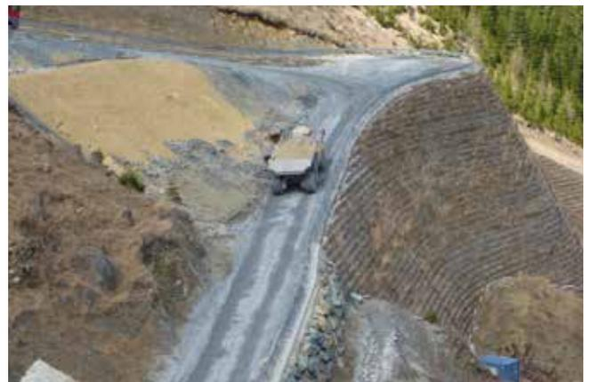
Figure 7: Adding quantities of soil to widen the access road resulted in a sudden rise in strain behind the structure
