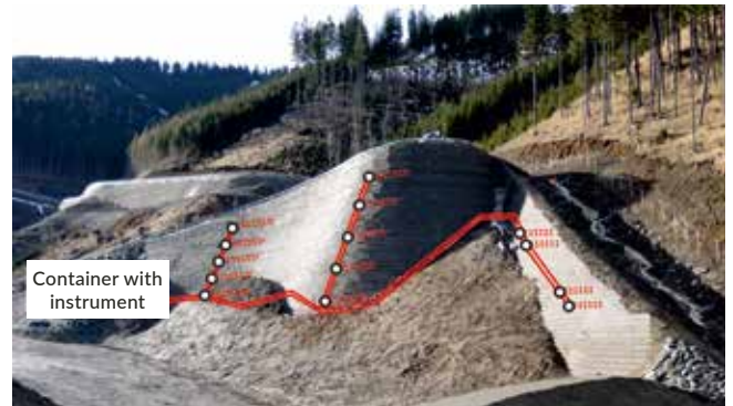
Figure 4: The geogrid and sensing cables were deployed within the earth retaining structure
