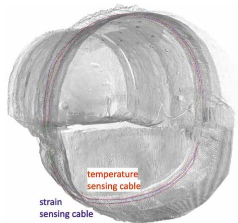
Figure 3: Position of sensing cables within the tunnel section, captured by laser scan
