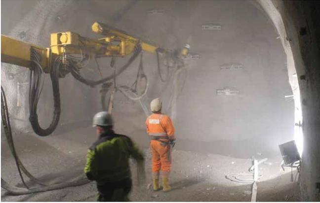
Figure 4: Shotcrete application to the top heading. Watch the video of the installation at <https://youtu.be/TYML8r3JI80>
