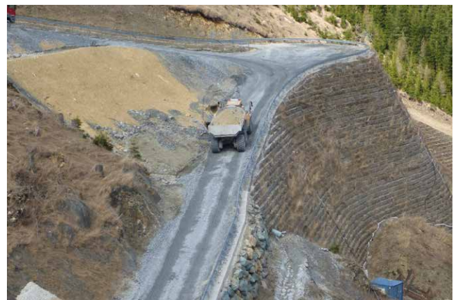
Figure 7: Adding quantities of soil to widen the access road resulted in a sudden rise in strain behind the structure
