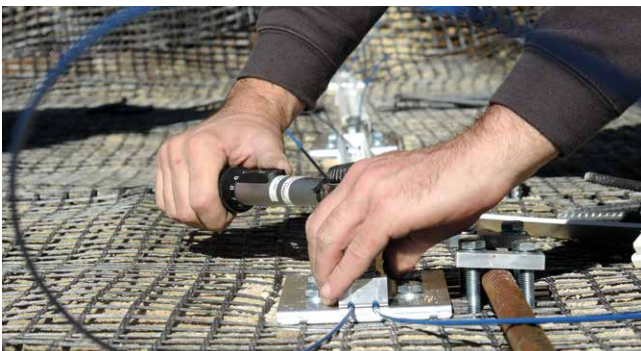
Figure 3: Attaching the fiber optic sensing cable to the geogrid
