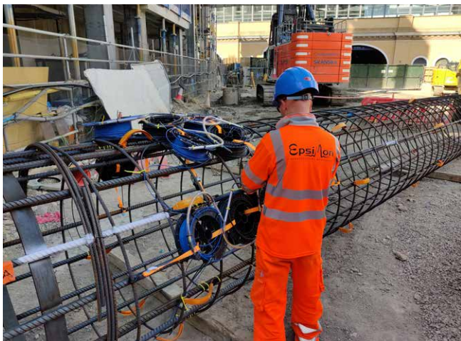
Figure 2: Pile cage instrumented with temperature and strain cables
